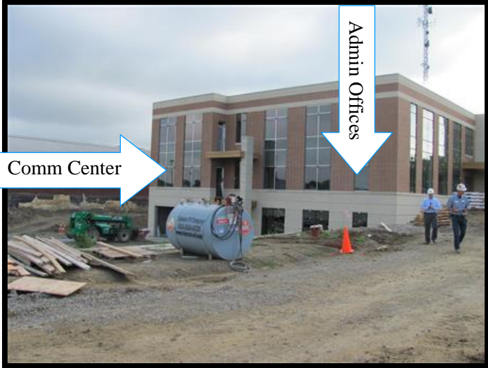
Southwest Corner of New Building
